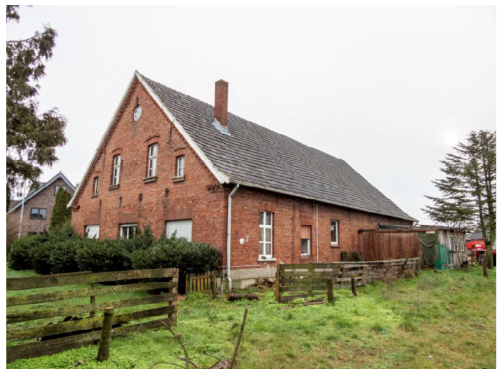
Blick aus West. (Foto: DSCN0017)
